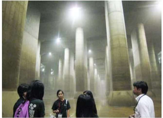
Punahou School Japan Wizards winning team tour the G-Cans massive underground concrete water storage facilities
